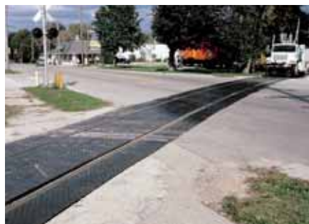
Fig. 1 PROTOTYPE CROSSING. Prefabricated crossings, like this rubber one, are the most common type in use today.
