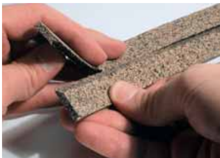
Fig. 1 SPLITTING CORK. Cork strips are perforated at an angle down the middle, and the two halves must be peeled apart. You need to sand the rough edges after laying.
