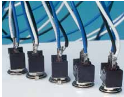
Marty prewired the toggles before installing them on the panel.
