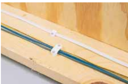
Fig. 11 WIRE STAPLES. Keep your wiring neat by using wire staples, which are available in many sizes.
