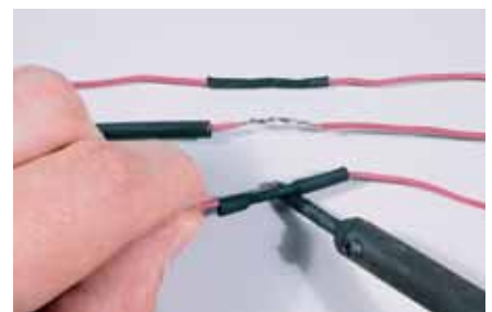
Fig. 7 HEAT-SHRINK TUBING. A finished joint is shown at top. Be sure to thread the tubing onto the wire before soldering the joint. Rub the tubing with the side of the iron, not the tip, to make it shrink.
